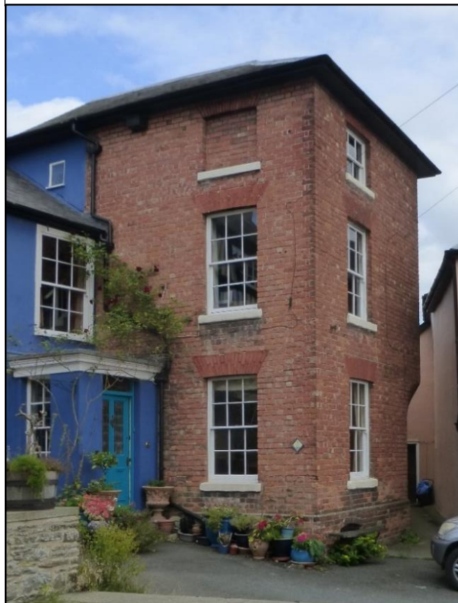
WELLFIELD HOUSE, Bull Street
