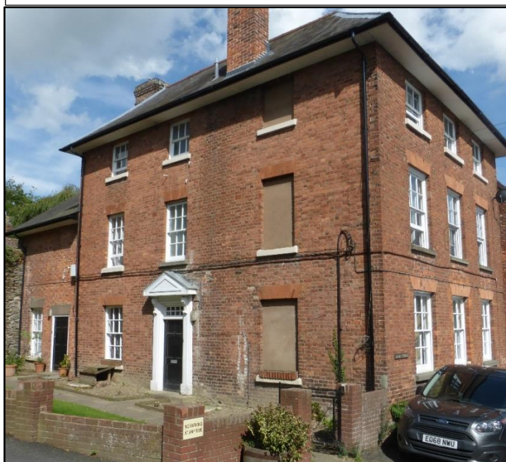
OLD BANK HOUSE, Market Square
