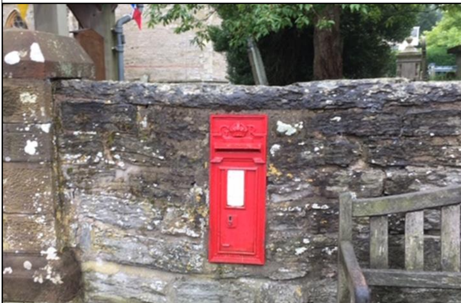
POST BOX, in the wall of St. John the Baptist Church, Church Bank
