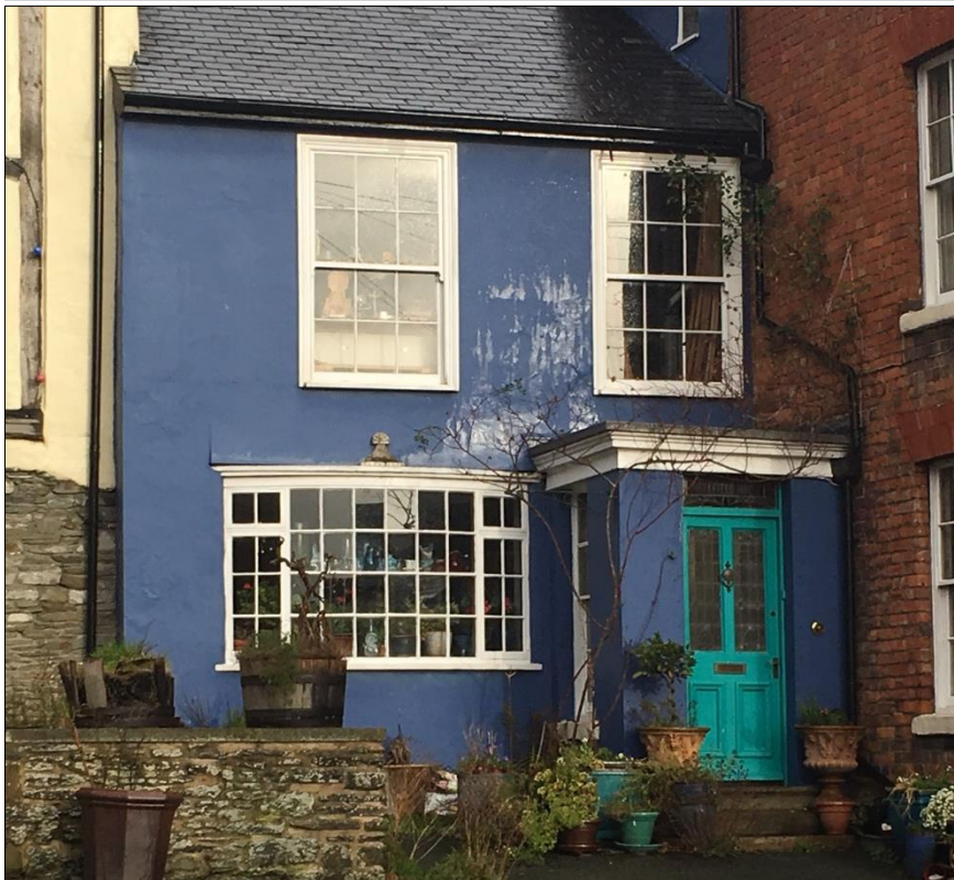
WELLFIELD HOUSE, Bull Street
