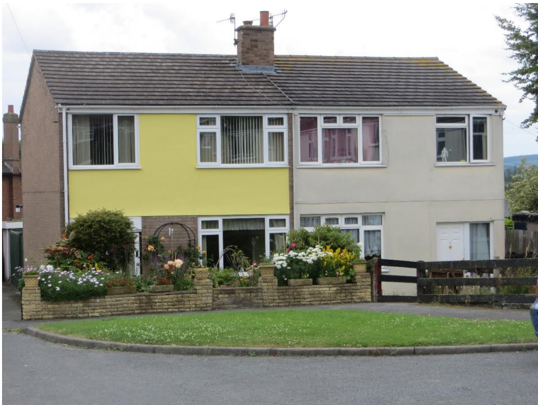
Painted insulation cladding
