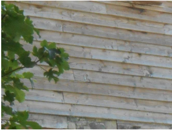
Timber cladding
