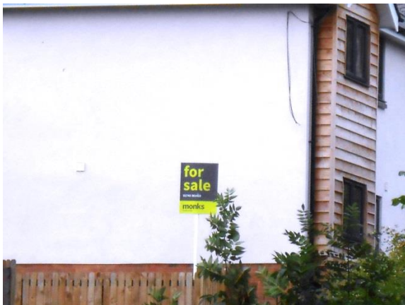
Render & timber cladding
