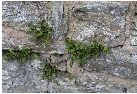
Wall rue growing on the boundary wall of no. 1
