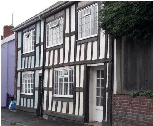
Half-timbered houses. Facades use traditional techniques
