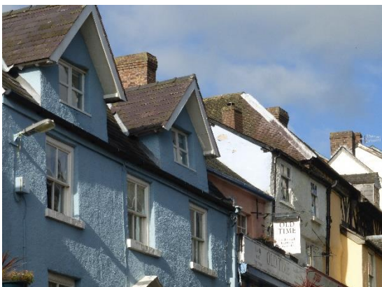
No. 27, the blue house stands proud of 29 and 31 at first floor level.
