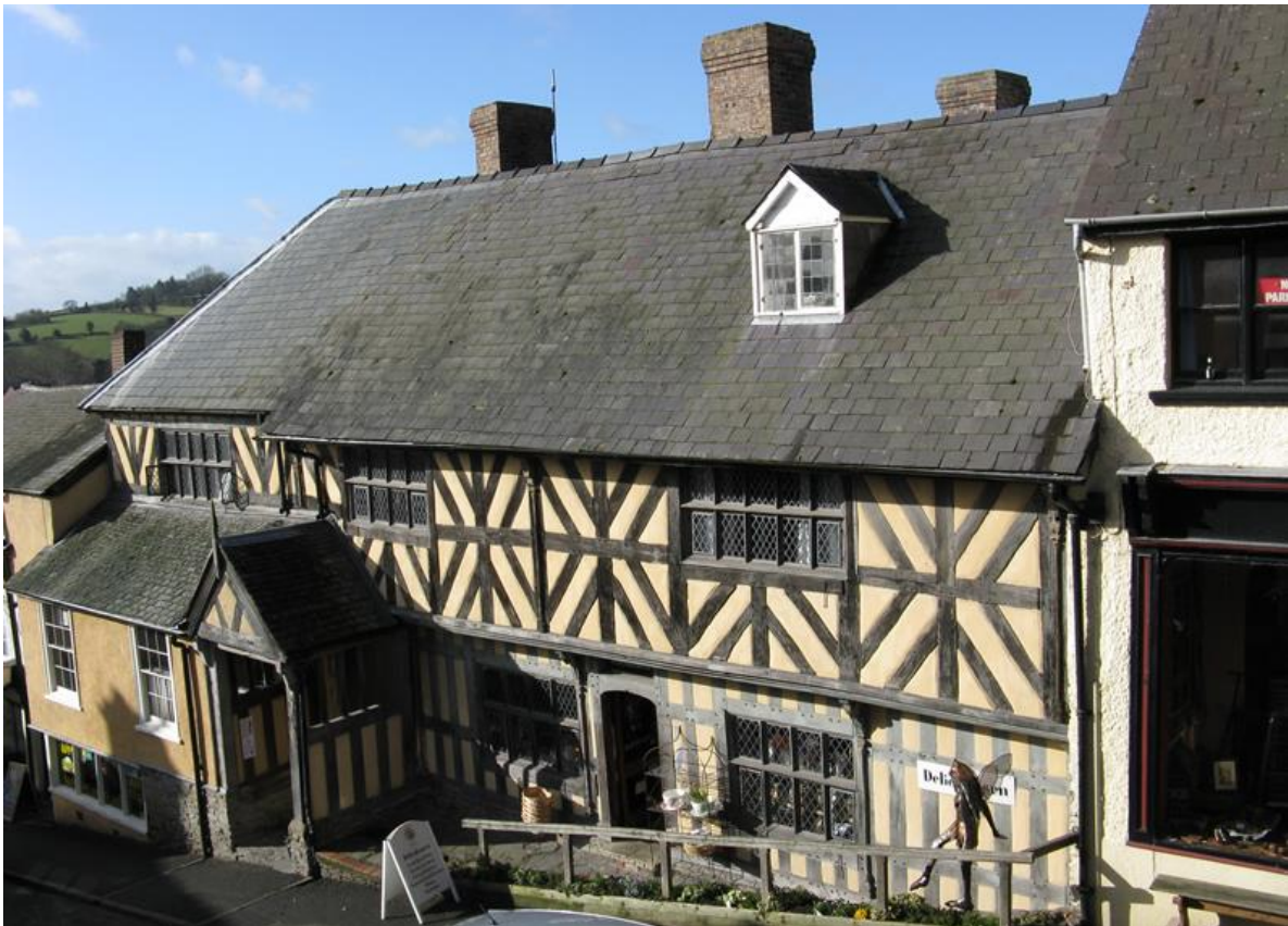
The C16 th Porch House
